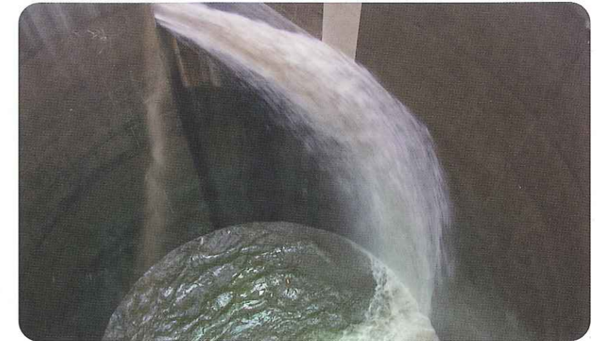
No. 5 bank (State of inflow)
